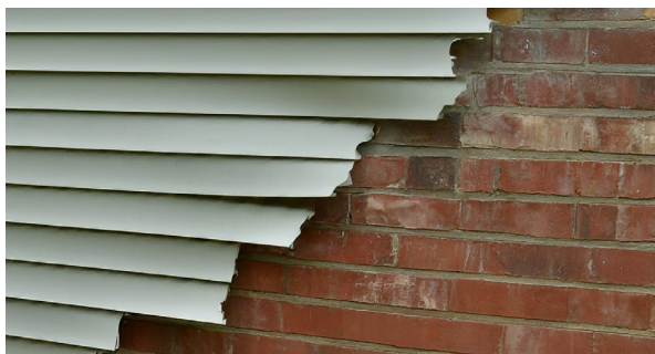
Removing vinyl to reveal brick below
