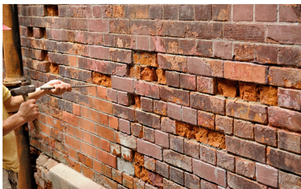
Repairing and repainting old brick walls
