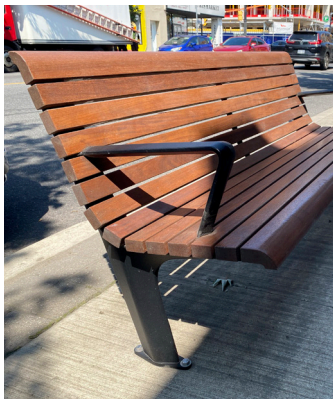
Durable benches and tree boxes. The wooden benches have just recently been sanded down and re-finished. The tree planters are anodized steel. Located in the Junction, Toronto.
